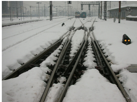
Typical Heated Points Systems using the RHT System - Milan, Italy.
